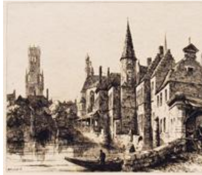
BRUGE Canal, with Tower of Boucherie in distance
